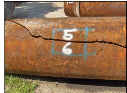
FKAA Transmission Main Replacement Key West, Florida
