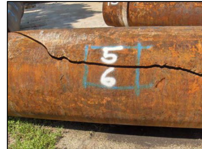
FCAA Transmission Main Replacement Key West, Florida
