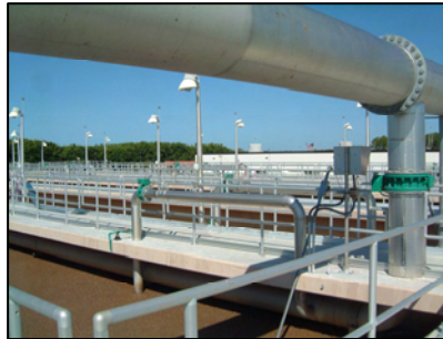
NCWRF Expansion Naples, Florida
